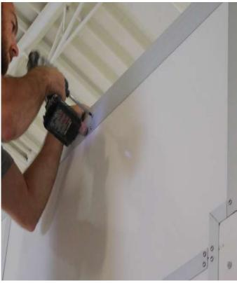
Secure Aluminum Channels to Ceiling Panels on all four sides with provided #10 sheet metal screws.
