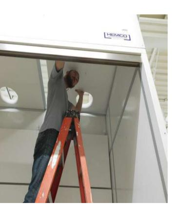
Install (Right Ceiling Panel C) into Aluminum channels.
