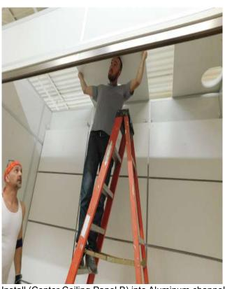
Install (Center Ceiling Panel B) into Aluminum channels. Install Aluminum channel between Ceiling Panels.
