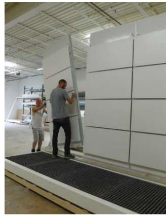
Attach Panel (Left Back Wall A) to (Center Back Wall B). Secure from back with provided #10 sheet metal screws.
