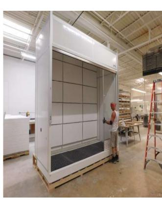
Install the (Sliding Door K) into the Door Frame .
