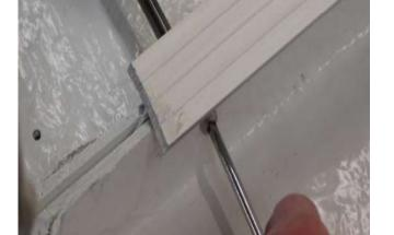
Install: Machine screws and locknuts to hold the ceiling panels together.
