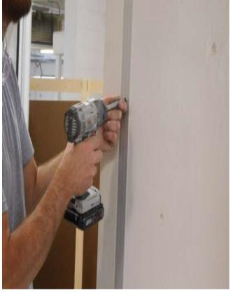
Secure from right and left sides with provided #10 sheet metal screws, and Bolts.
