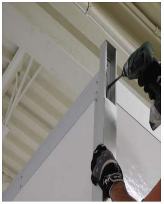
Install Left and Right (Electrical Chases), to front corners of hood. Secure with provided #10 sheet metal screws.
