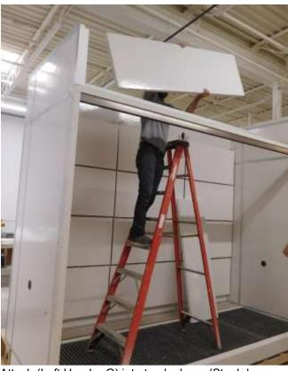
Attach (Left Header G) into track above (Steel door frame I).
