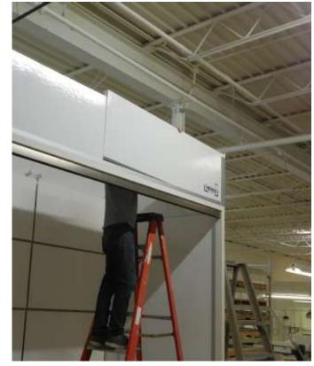
Attach (Right Header I) into track above (Steel door frame I) insert aluminum channel between headers.
