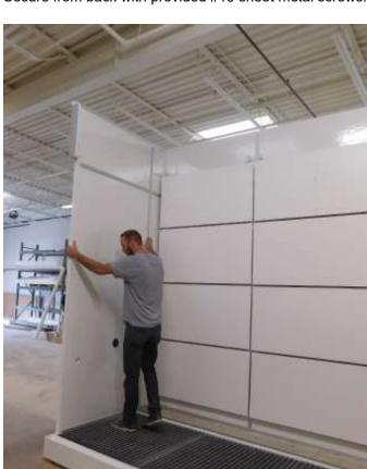
Attach Panel (Left Wall H / F) to (Left Back Wall A). Secure from back with provided #10 sheet metal screws.
