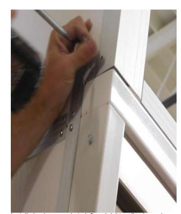
Install aluminum angle to left and right walls above door frame. Secure with provided #10 sheet metal screws.
