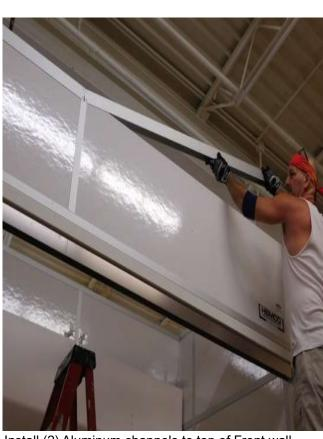
Install (2) Aluminum channels to top of Front wall.
