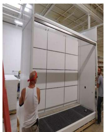
Move (Steel Door Frame) into position.
