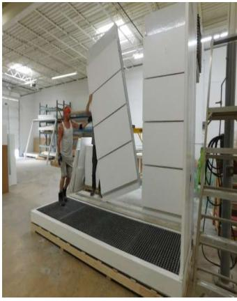
Attach Panel (Center Back Wall B) to (Right Back Wall C). Secure from back with provided #10 sheet metal screws.
