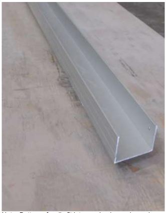
Note: Bottom of walls fit into an aluminum channel.
