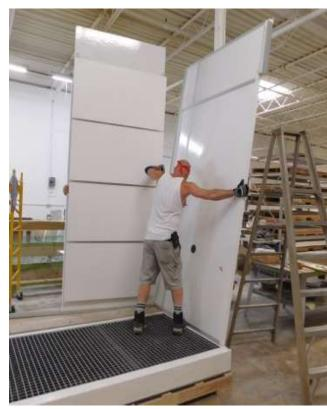
Attach Panel (Right Side Walls D / E) to (Right Side Back Wall C). Secure From back with #10 sheet metal screws.
