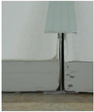
Aluminum channel shown in position between ceiling panels.
